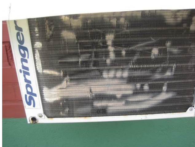
Figure 32: Major Deformities in Heat Exchanger Ribs
