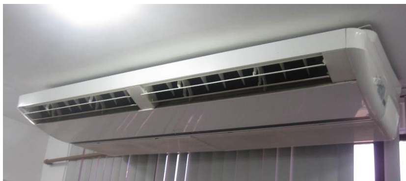
Figure 18: Installed Ceiling Split Unit
