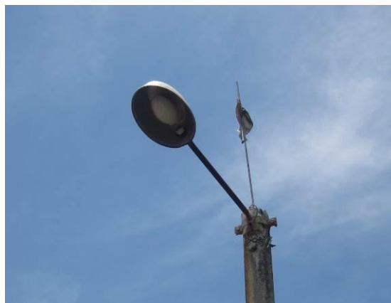
Figure 26: Installed Mercury Vapour Lamps
