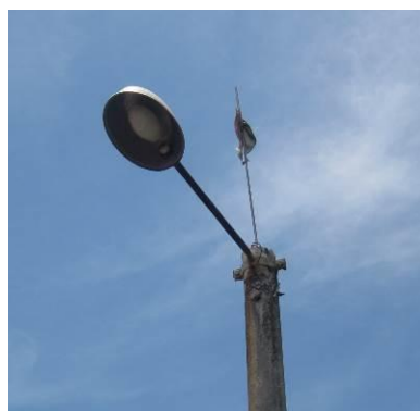
Figure 17: Installed 250 W Mercury Vapour Lamps
