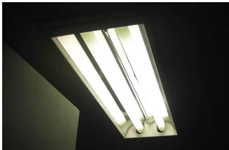
Figure 24: Installed T12 Lamps
