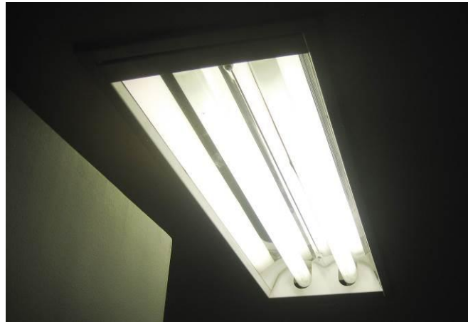
Figure 15: Installed T12 Lamps
