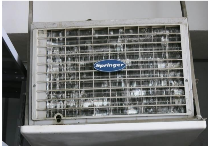
Figure 30: Major Deformities in Heat Exchanger Ribs
