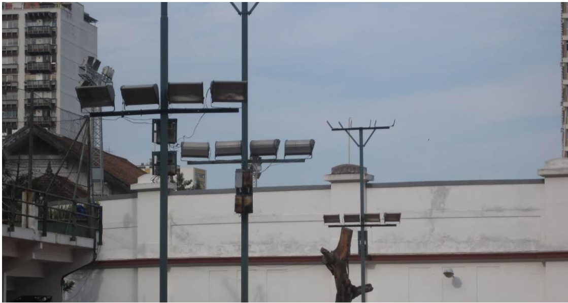
Figure 16: 400 W Mercury Vapour Lamps Installed in Tennis Courts.
