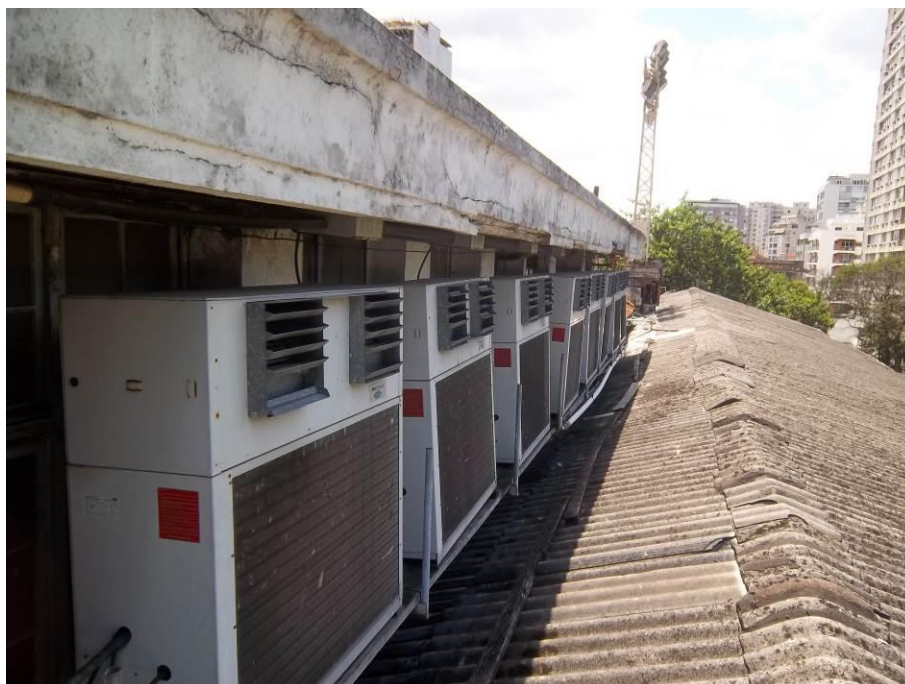
Figure 21: Condensing Units of Multi Split Units
