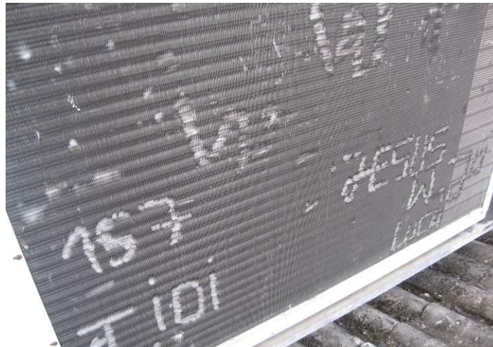
Figure 31: Major Deformities in Heat Exchanger Ribs
